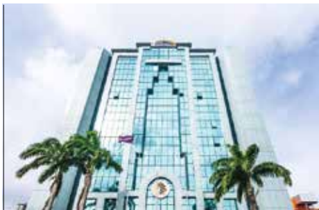
The headquarters of Africa Re in Victoria Island, Lagos.
